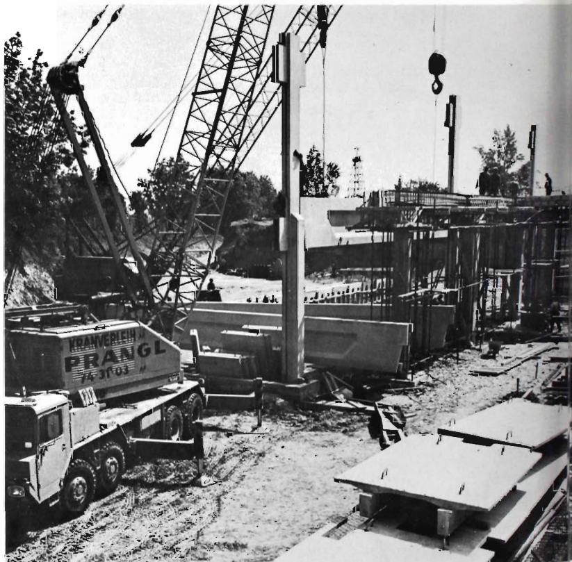
Fig. 9 To simplify construction most of the buildings in the Zentrum Wien complex utilized a system of reinforced-concrete girders and standardized supporting pillars which latch together somewhat like a giant erector set.
