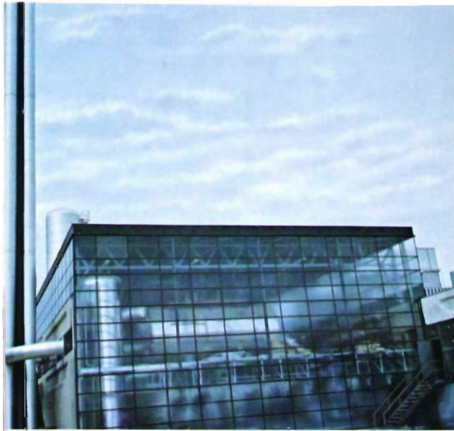
Fig. 30 Power source for the whole complex is in this building—called "Energy Central". Here are located main air conditioning units, emergency generators, boilers, etc.—and all power control. A fuel oil storage tank stands just behind this building.
