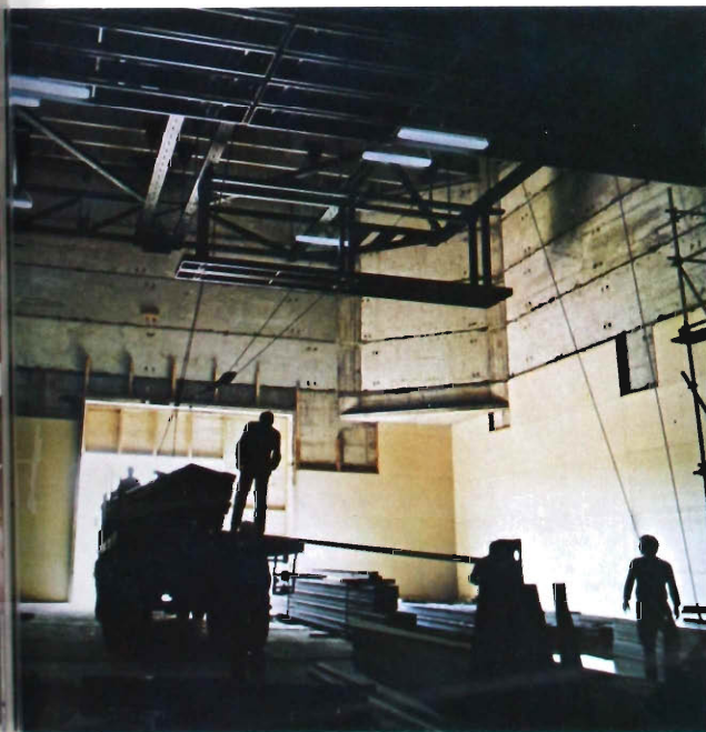
Fig. 17 The roofs of the studios are made up of T-shaped reinforced-concrete beams. The vertical sections of these beams provide rigidity and a convenient place for attaching the hangers which support the overhead structure.
