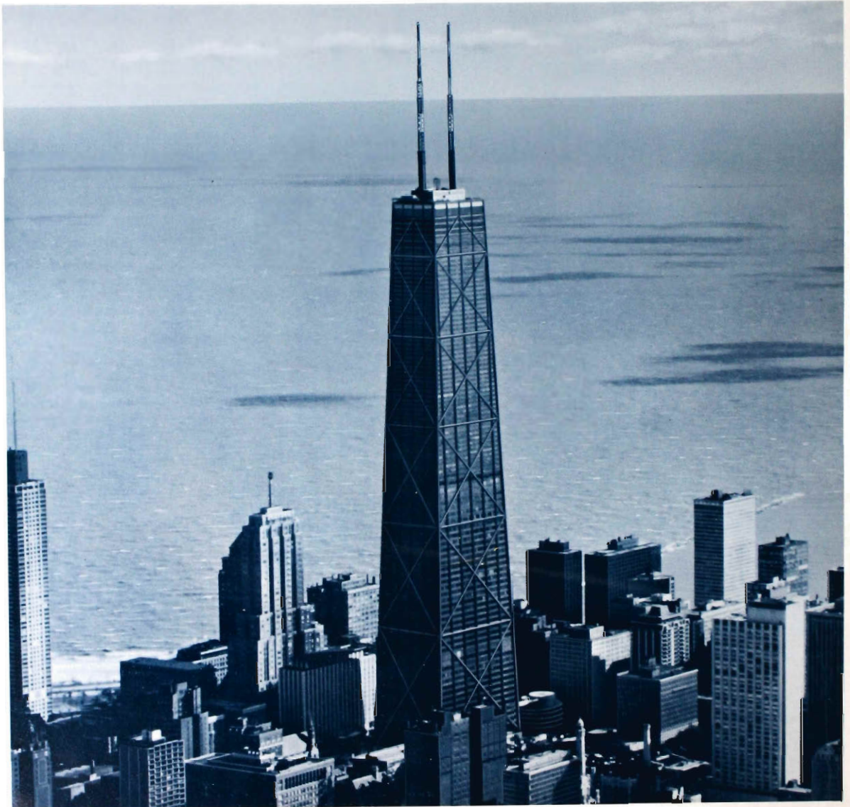
John Hancock Center dominates Chicago skyline.
